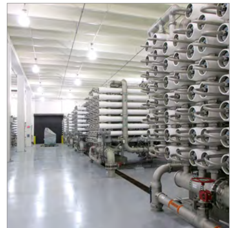
Figure 1: Reverse Osmosis/Nanofiltration
