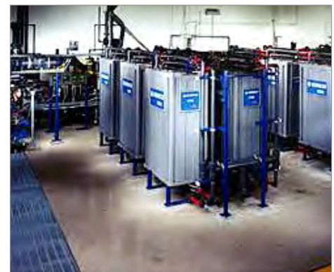
Figure 2: Electrodialysis Reversal (EDR)
