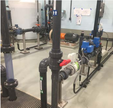
Photo shows a fully automated neutralization system
