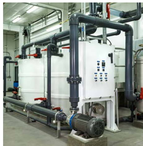
Photos show typical packaged CIP systems for NF/RO
