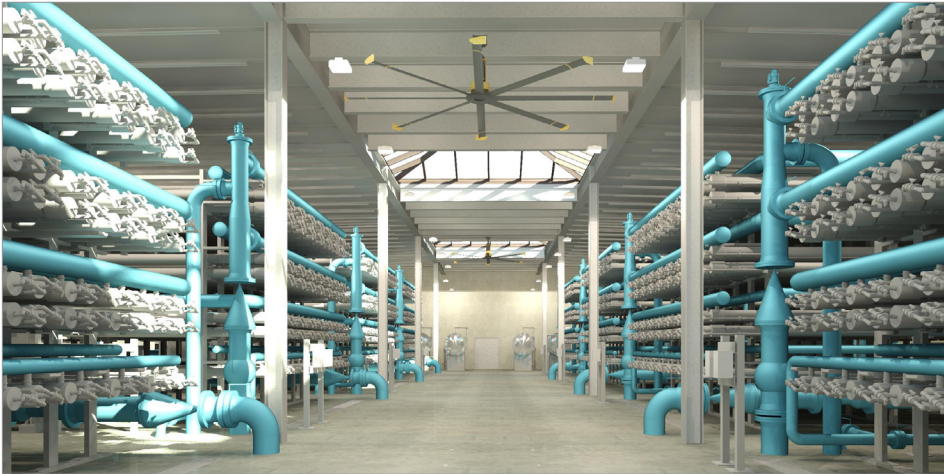
Figure 3: PFAS Removal Facility Under Construction in Brunswick County, NC
