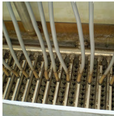
Figure 5: Example of immersed (submerged) membranes
